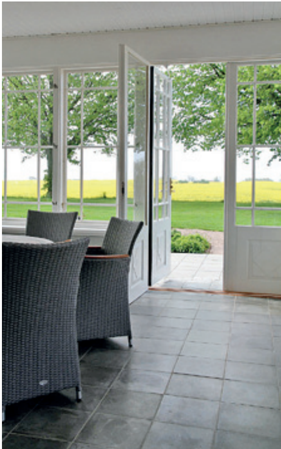
Concrete tiles treated with natural Linseed Oil Wax.
